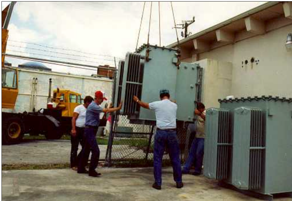
Figure 4a. Photo, IOT system outdoor components: workers move 36 kV beam supply into final position.
